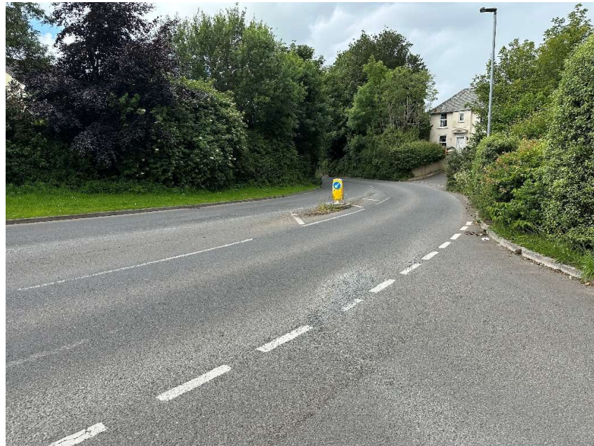
A379 Church Street at Lanveoc Way, No Footways – Aprica Image
