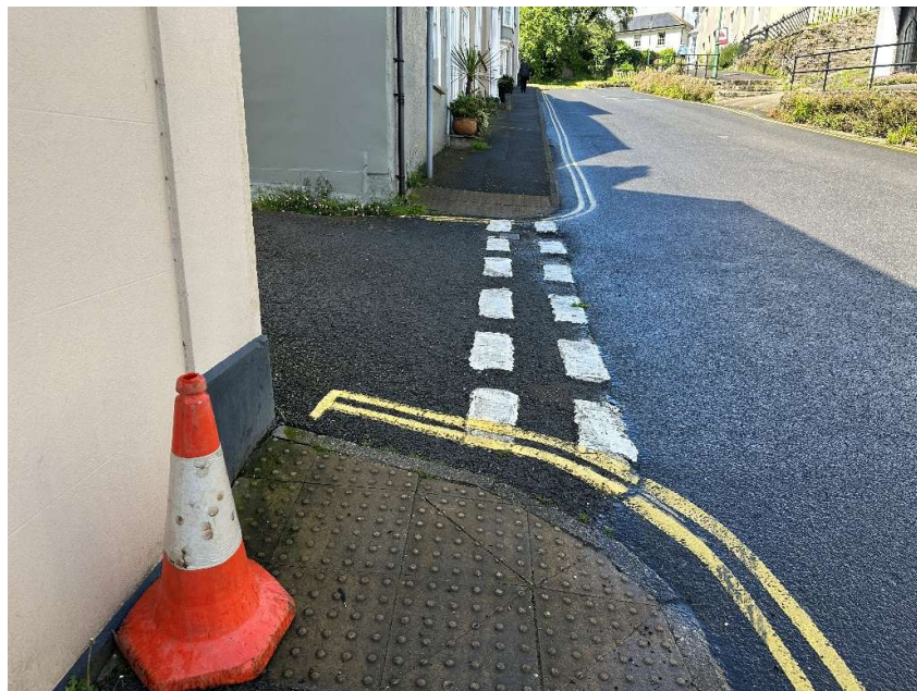
Church Street Narrow Southern Footway (Terminating) - Aprica Image
