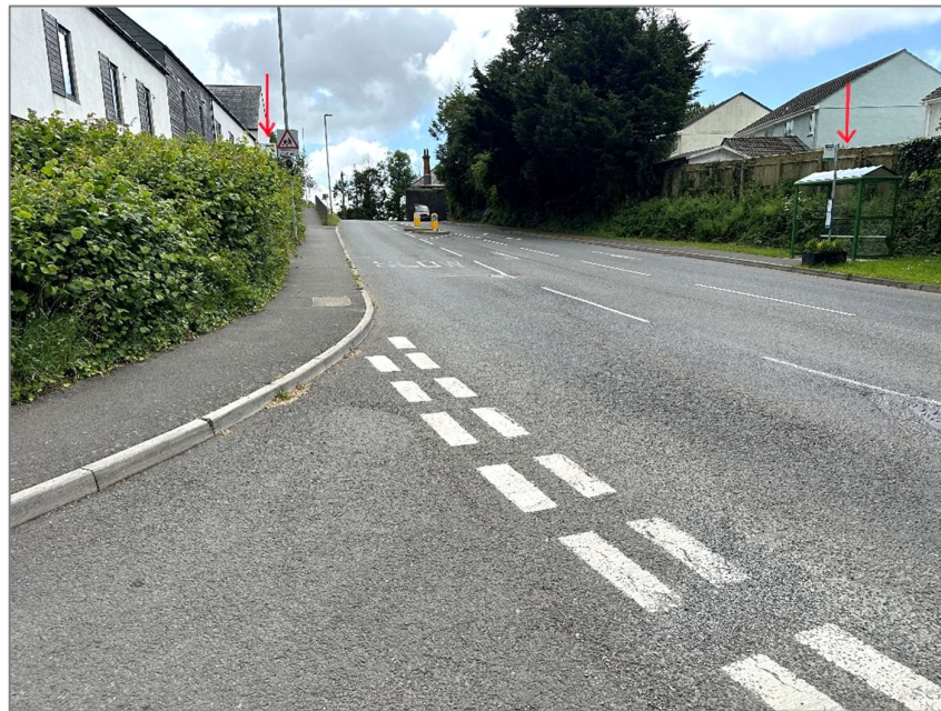
Bus Stops (Arrowed) Failing Current Standards - Aprica Image
